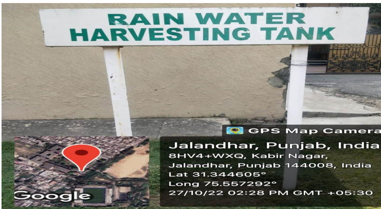
Rain water harvesting tank installed in the DAVIET Campus
