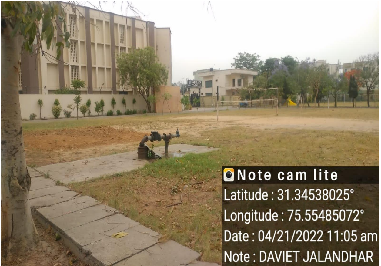
Water pumping and withdrawal facilities available within the Institute
