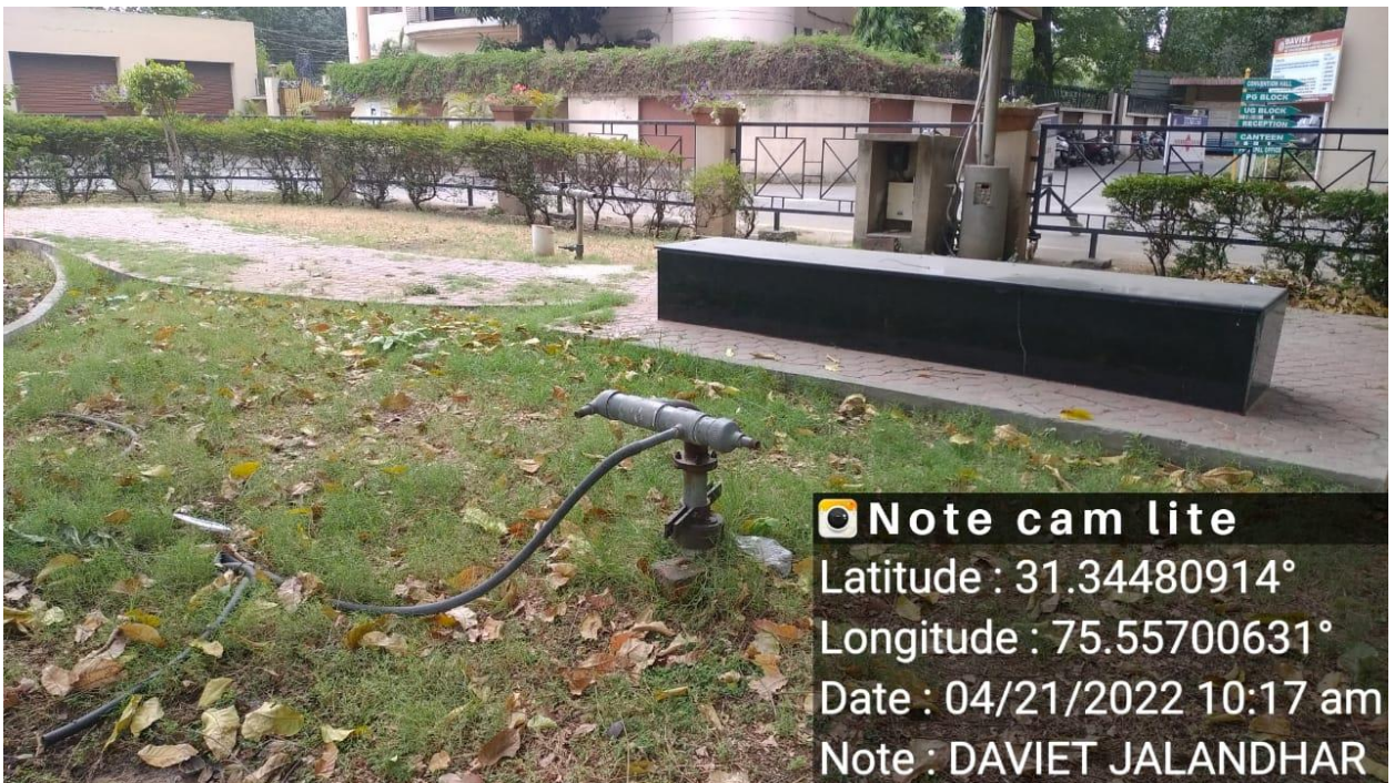
Water pumping and withdrawal facilities available within the Institute
