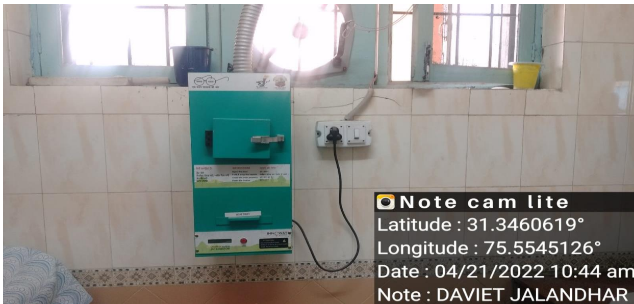
Incinerator (used for disposal of biomedical waste) in the in the Girl hostel washroom
