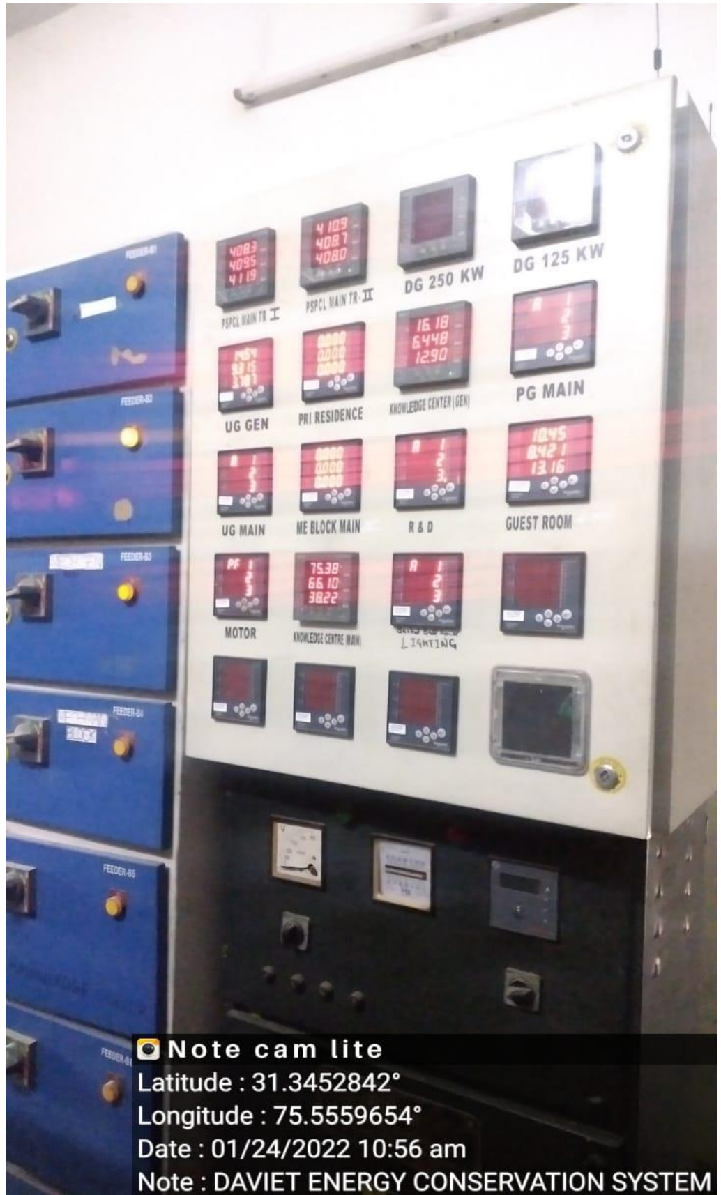
MFM Schneider Smart meter for the Sensor based energy conservation systems (3 no.) installed in DAVIET, Jalandhar
